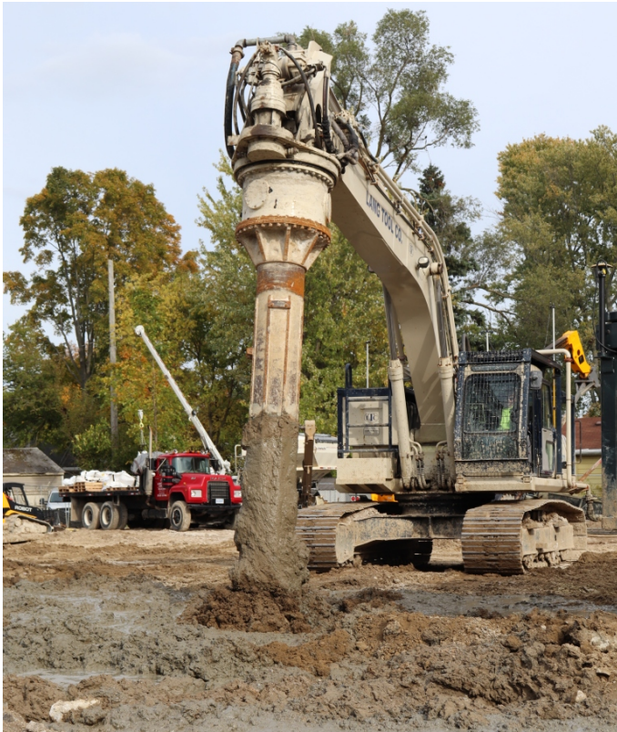
Dual Axis Blender mixing the last cell on the Kent Cleaners Project.
