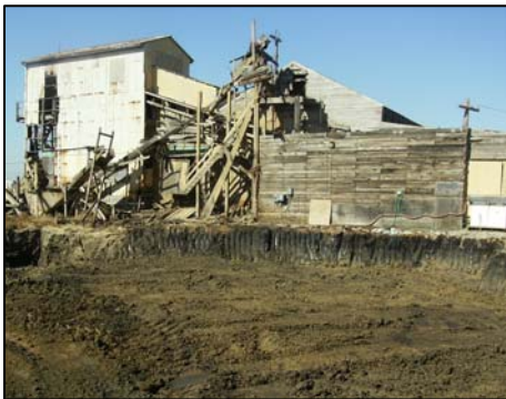
Figure 1. Former Industrial Facility
